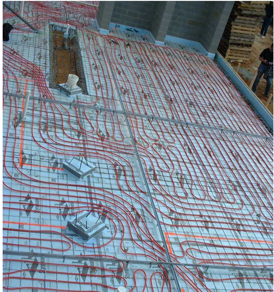
Fig. 09 Radiant floor piping installation
