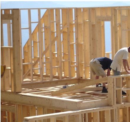
Fig. 03 Timber frame construction
