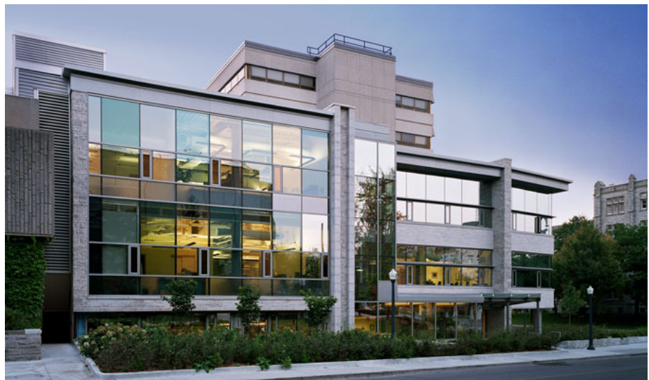
Fig. 11 Integrated Learning Center at BeamishMunro Hall
