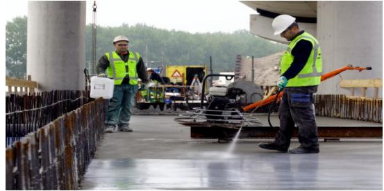
Fig.1.3 Water sealant layer over the bridge using seaweed extract
