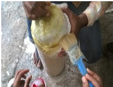
Fig.16: Dome being attached to the cylindrical portion
