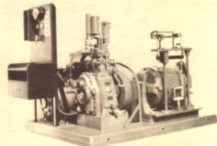
This is the first CFR dynamometer unit built for the U.S. Army. Circa 1931. This unit permitted testing of fuels at various horsepower.
