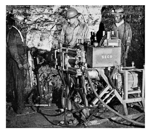
Figure 7. Drilling coal specimens for properties testing
