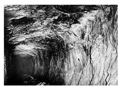
Figure 10a. Square tunnel in quartzite remote from mining activities. Depth of 9,500 ft. below surface in a South African gold mine
