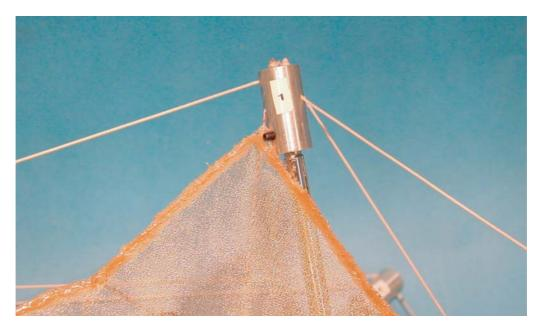
Figure 7.13: Cylindrical joint fitting with grub screw.
