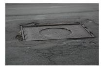
Figure 11: Severely sunk-in manhole, with eroded edges. This generated a pothole detection.
