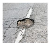
Figure 10: Typical small pothole with missing pavement.
