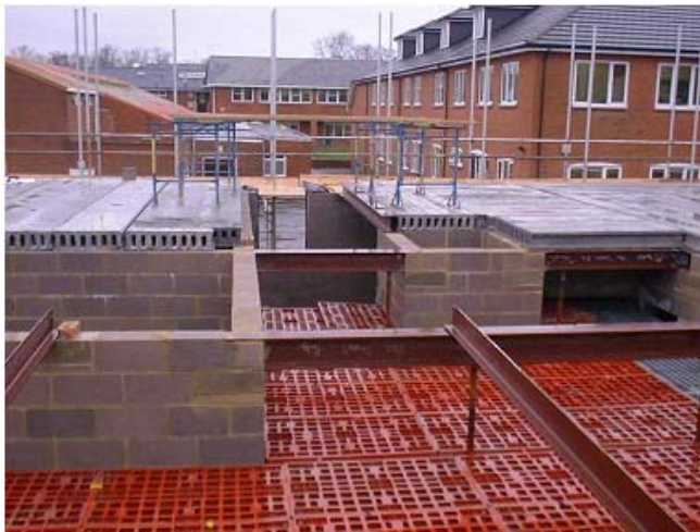
Figure 4-2. Metal decking system. (A) View of a Metal decking system during steel or timber erection work and (B) Metal decking system during masonry work (Source: Health Safety Executive Research Report 302, 2003).
