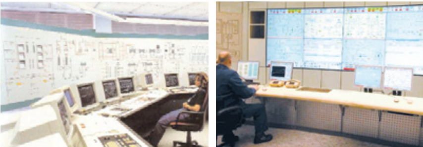
Figure 4.10 – Control room of ‘Jämschwalde 6x500 MW’ plant : Before (left) and after (right) a DCS modernization. Source: ABB Industrial IT for Power Plants.
