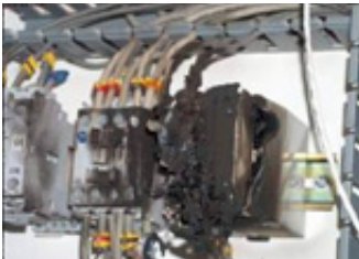
Figure 3.7- Harmonics-induced damage, (ABB Kurt Schipman , 'Active Filter Savings', 2008)
