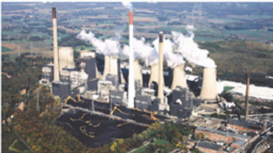
Figure 5.4 – ABB AG Power Technology Systems, 2006
