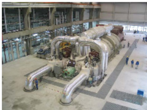
Figure 5.7 – Turbine Generator unit photo, (ABB Solutions for Fossil Fuel Power Plants brochure, 2007)
