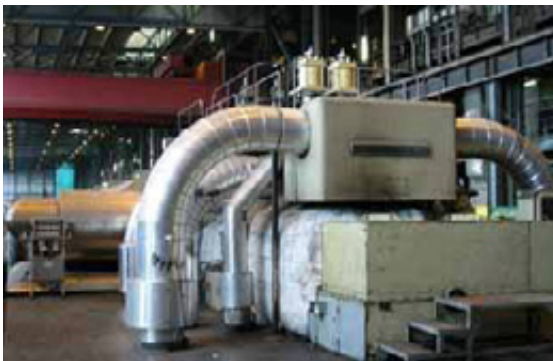
Figure 5.9 – CPT Blénod Power Plant Units 3 &4, EDF, France
