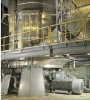
Figure 5.19 – Coal pulverizer with motor, (ABB Motors, 2006)
