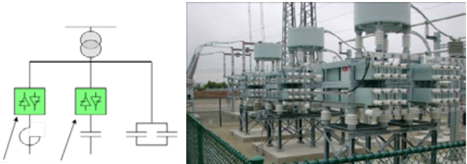
Figure 3.3 – SVC switches for reactance (left) and capacitance (right), (ABB Grid Systems,2009)
