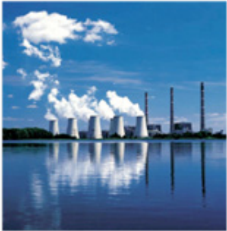
Figure 5.17 – Condenser cooling system towers, (ABB Ltd., Power Generation Unit, 2006)
