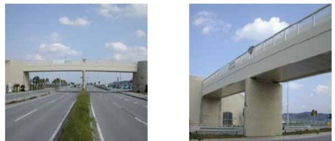
Fig – 8 Pedestrian Bridge in Okinawa, Japan made of Hybrid Composite
